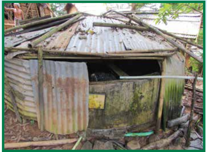
Present condition reveals the GFS to be still well-functioning
