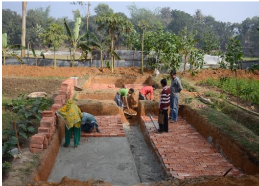
(a) Drying beds – masonry work
