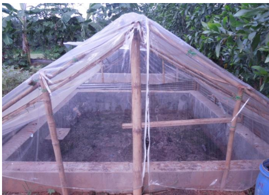
(c) Drying bed 1 with plastic cover
