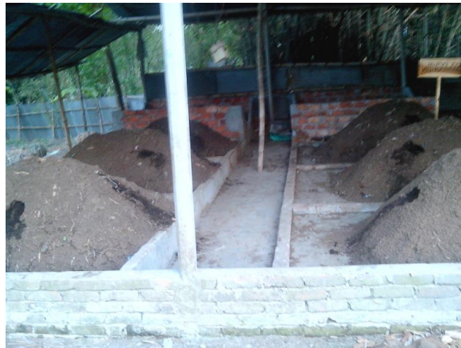
Figure 14 Photograph showing windrows 4-6 on the left hand side
