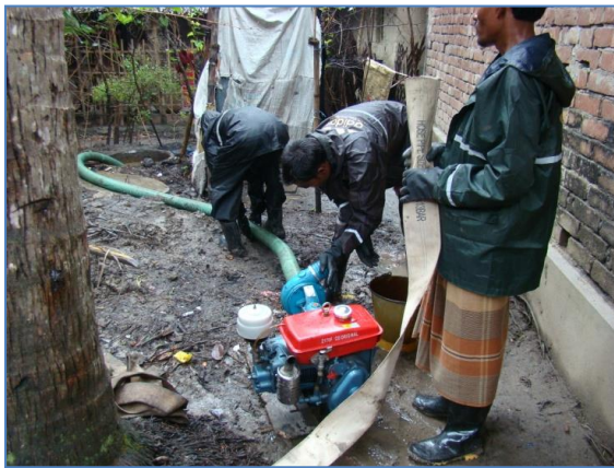
(c) Diesel pump
