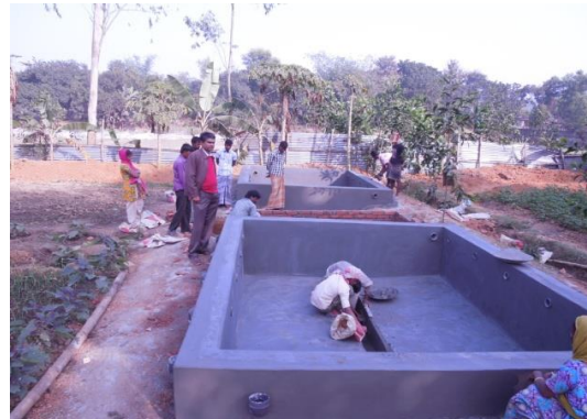
(b) Drying beds – plastering work
